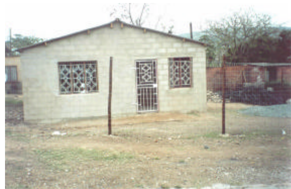
Figure 12: new four room houses in KwaMashu.
