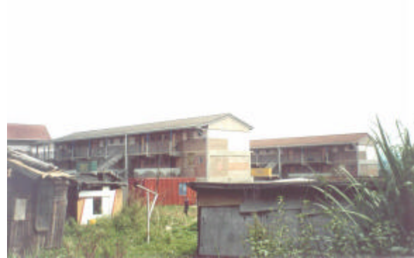
Figure 4: New hostels in KwaMashu A, also with informal shacks in between.
