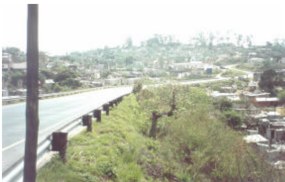
Figure 11: Overgrown area next to regularly targeted intersection. The topography also contributes to a lack of opportunities for surveillance.
